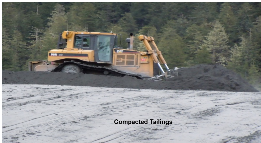
Photo 3-12, Spreading and Compacting Tailings
