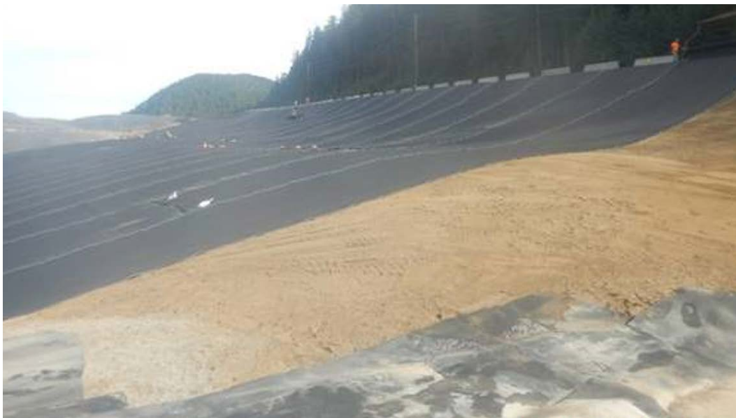
Photo 3-6, Placement of Synthetic Liner
