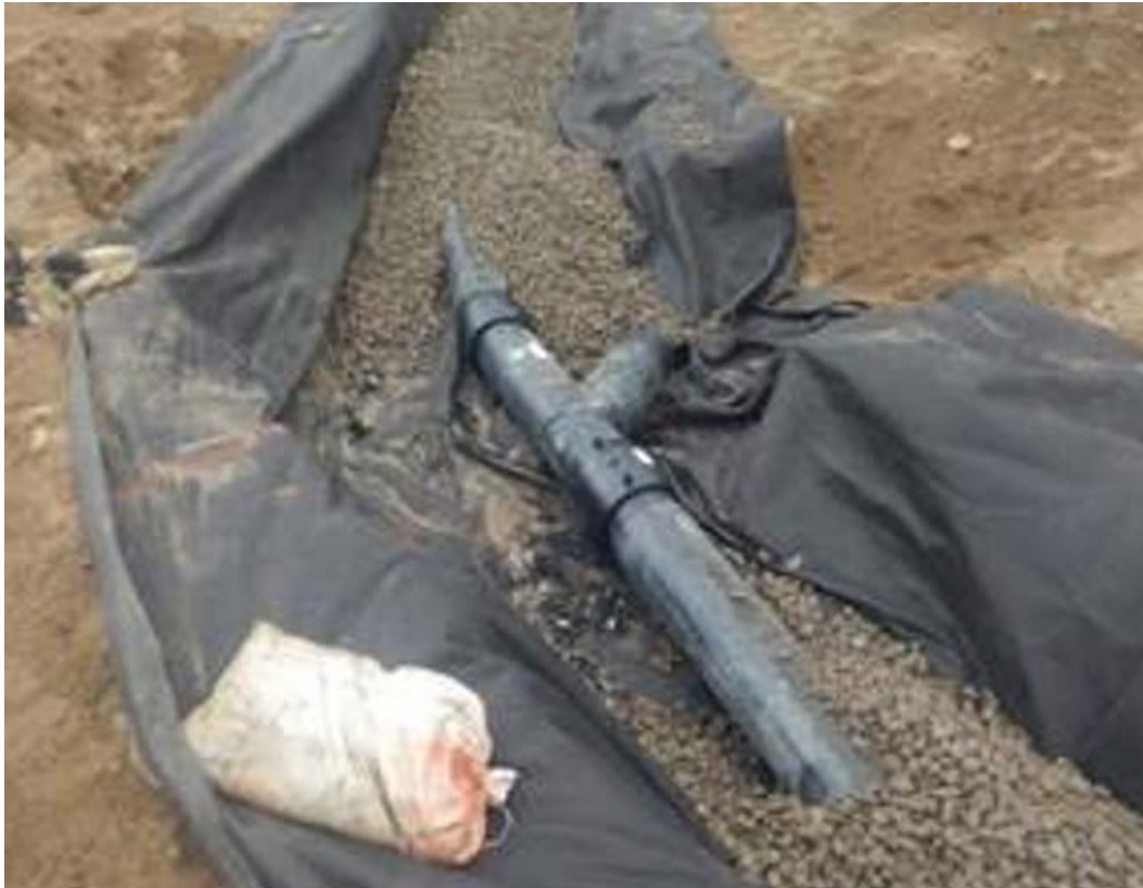
Photo 3-6, Placement of Synthetic Liner
