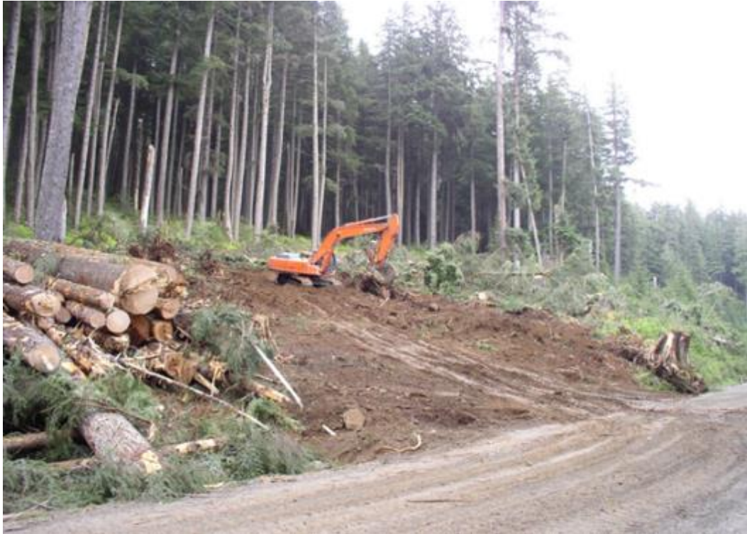
Photo 3-2, Foundation Preparation and Peat Removal as Necessary
