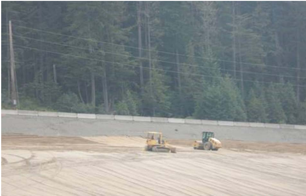
Photo 3-4, Placement and Compaction of Bedding Layer
