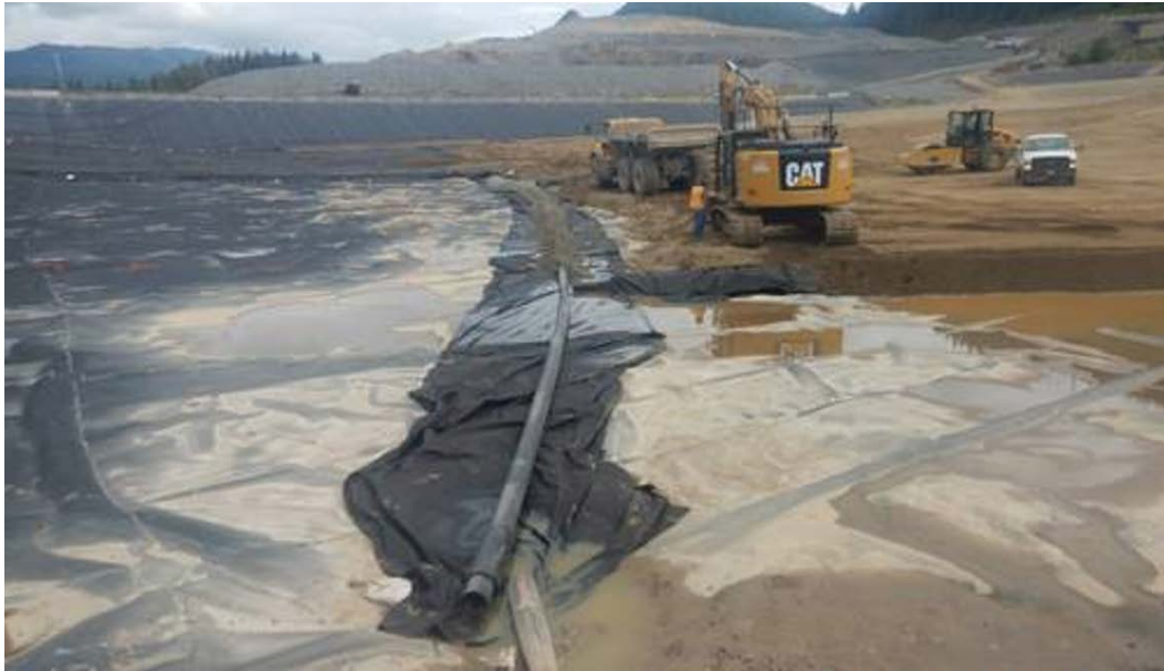
Photo 3-8, Placement and Compaction of Service Layer
