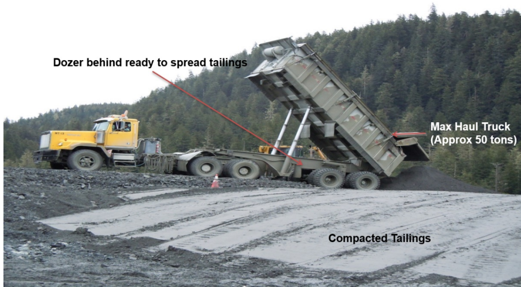
Photo 3-12, Spreading and Compacting Tailings
