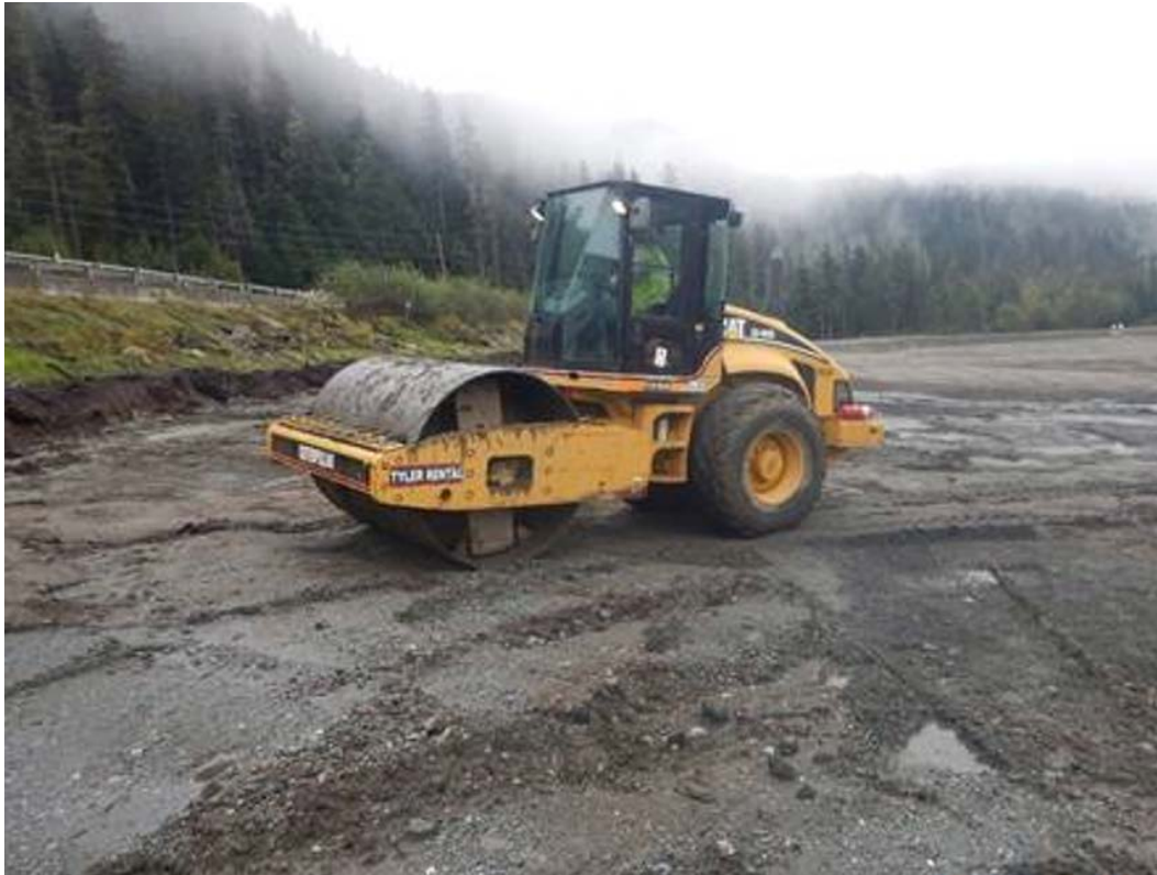
Photo 3-4, Placement and Compaction of Bedding Layer
