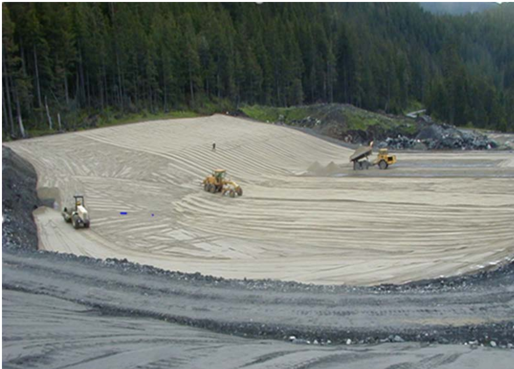
Photo 3-8, Placement and Compaction of Service Layer
