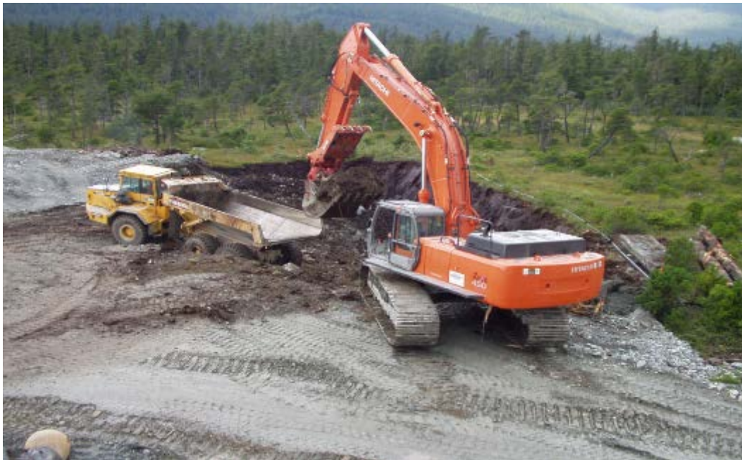
Photo 3-2, Foundation Preparation and Peat Removal as Necessary
