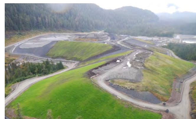
Dry-stack method of tailings management at the Greens Creek Mine in Alaska.
