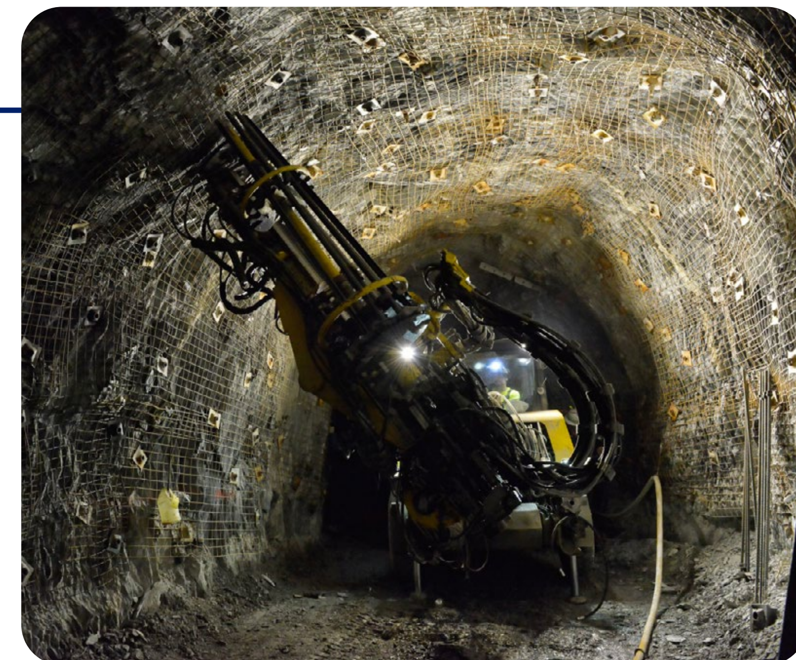
Underground rock bolter, Lucky Friday mine
