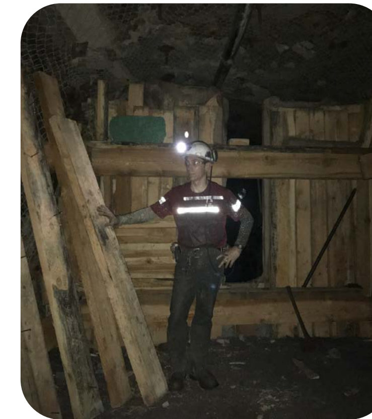
Chris building a sand wall at Lucky Friday around 2018
