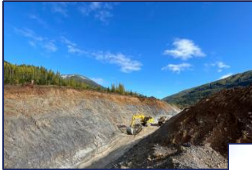
Pond 5 tailings project
