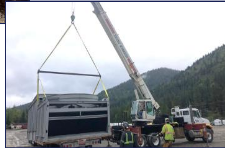
Surface Cooling Project
