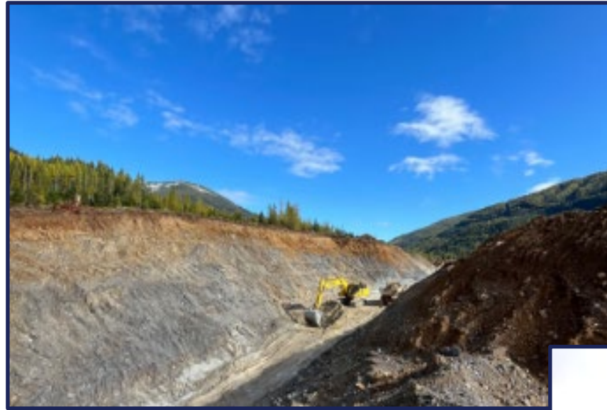
Pond 5 tailings project
