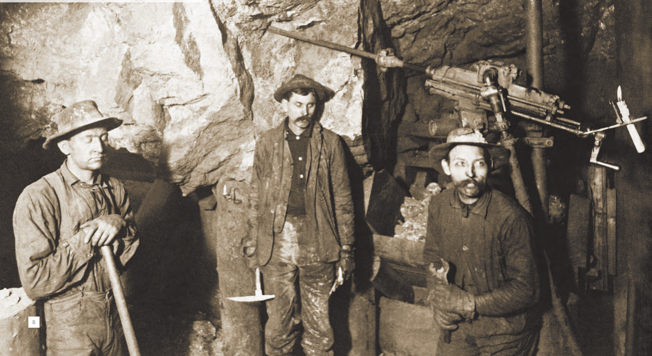
Three miners pose with hand tools in front of a jackleg drill lit by a single candle. They're underground at the original Hecla mine in Burke, Idaho, which yielded more than nine million tons of ore before closing in 1944.
