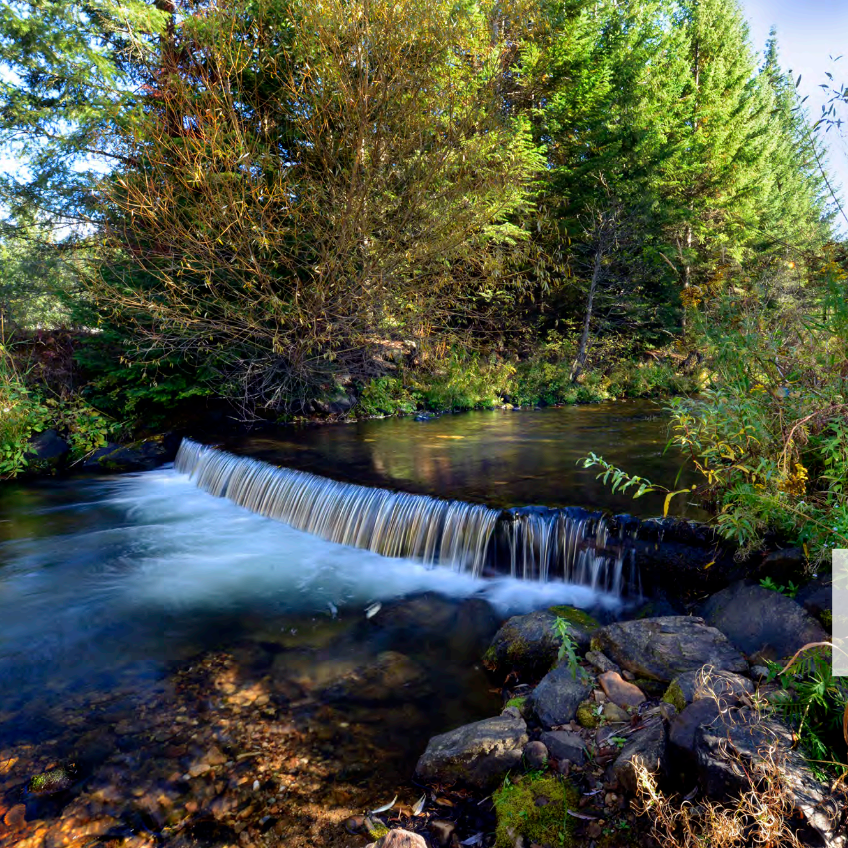
A Hewitt ramp near the Lucky Friday mine improves fish habitat by creating plunge pools and slowing and aerating the stream. The area is part of an expanded riparian habitat for moose, beaver, frogs, and wetland plants.
