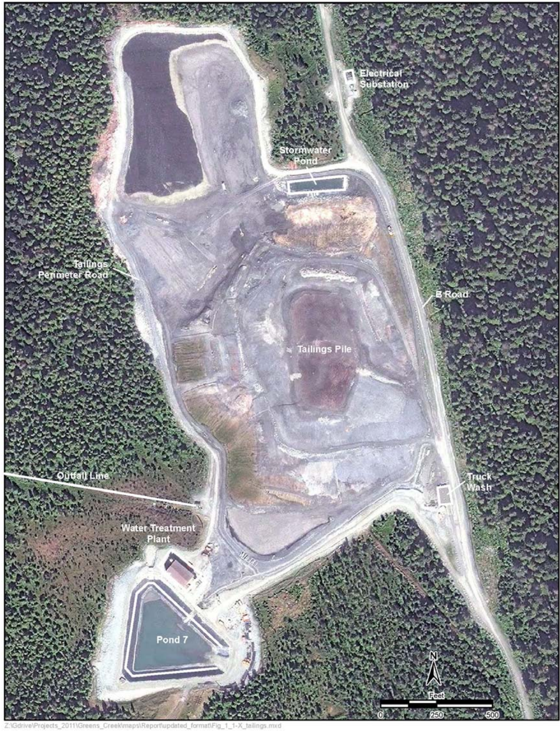
Figure 1.1-3. Greens Creek Tailings Facility (2009).
